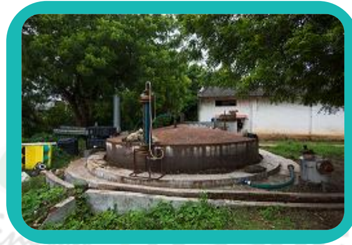
Community based Biogas Plant (25-1000 m 3 )
