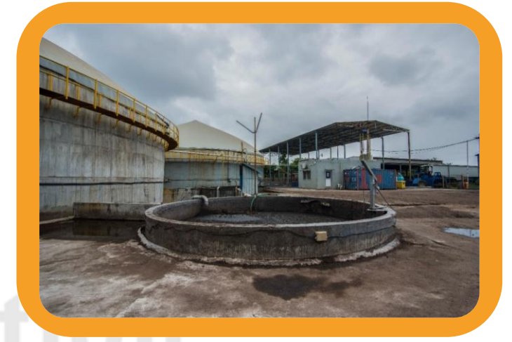
Large Scale Biogas Plant (>2500m 3 )
